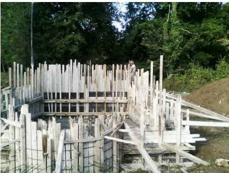
In preparation for concrete
