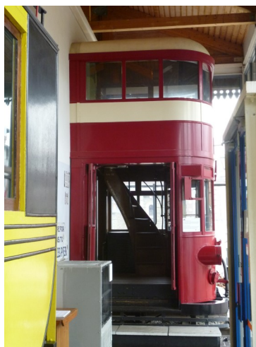
Cab front jig under construction in Alikes
