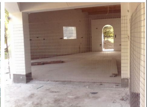
Awaiting underfloor heating
