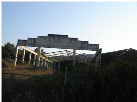
“New main railway construction near Varipatades”
