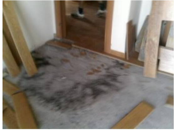
'The old floor was ill-fitted'
