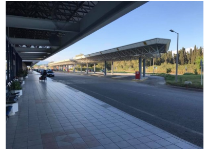
Early Doors at Corfu airport, photo courtesy of Jon Whitaker
