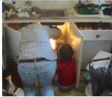
'Mending the sink drain u-bend in the utility room' <
