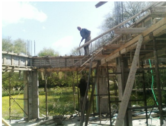
1 The team is in to pour concrete for the main ring beam
