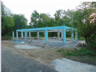
1 The team is in to pour concrete for the main ring beam
