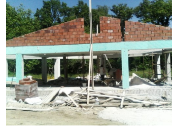
6 Bricking up to get the roof on
