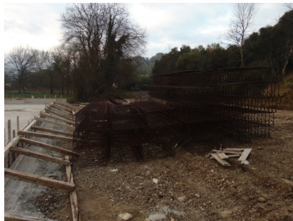
Steel delivery for new villa
