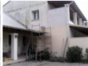
Scaffold in place for chimney work
