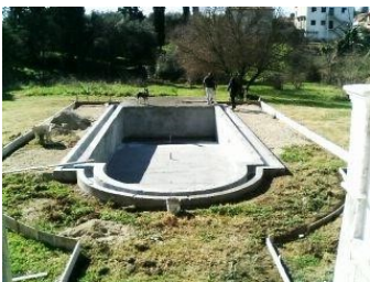
Formwork from the villa
