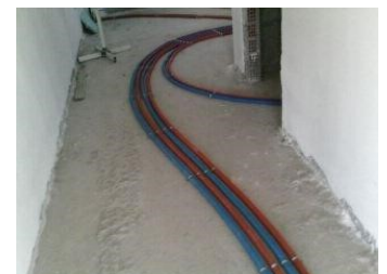
Pipes for central heating
