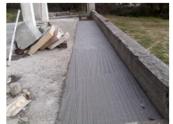
Getting ready for surfacing
