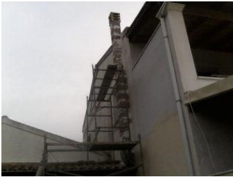
Building a chimney
