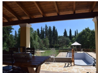
Pool ready to fill
