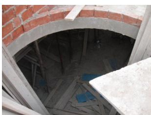
Forming of a spiral oak staircase
