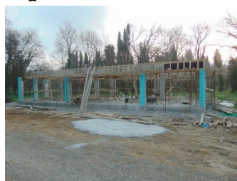
New villa under construction
